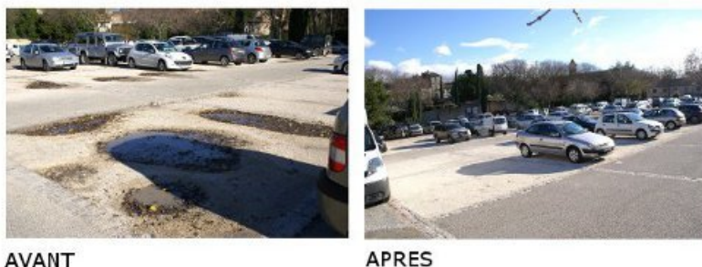
Parking des Cordeliers, Uzès
